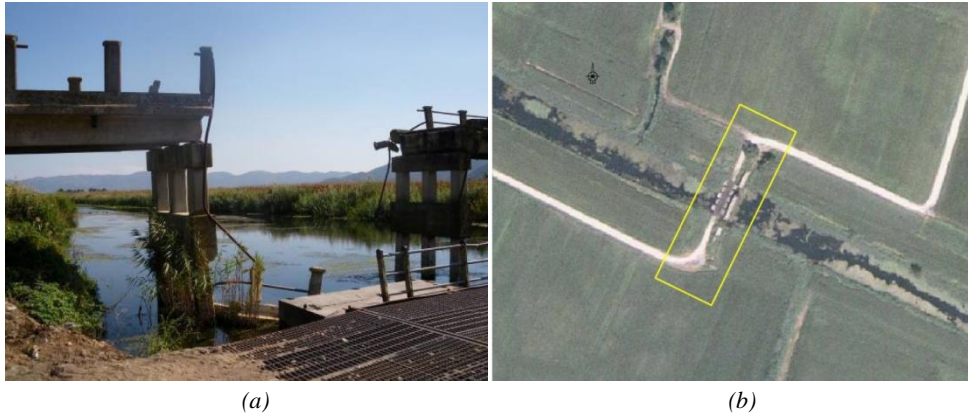
Figure 1. (a) The existing bridge, and (b) the location of the project
