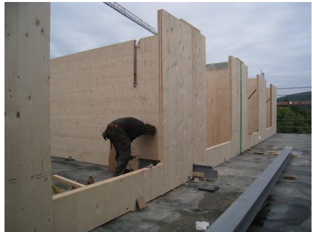
Figure 5: Plywood wall elements assembly, Kierling, Austria © Architekturbüro Reinberg
