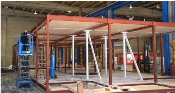
Figure 4: Offsite 3D modules manufacturing, Barcelona, Spain © La Casa Por El Tejado
