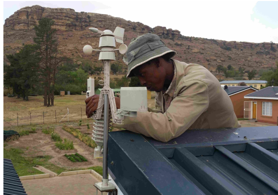
Figure 5. Weather station installation at LDF health clinic by STG International staff (Makoanyane Khakhanyo)
