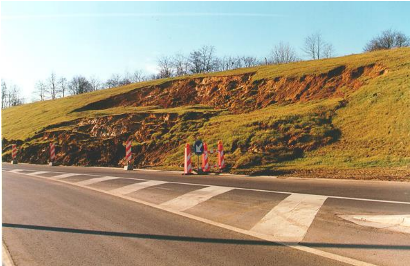
Human-made slope along E42 exit road
