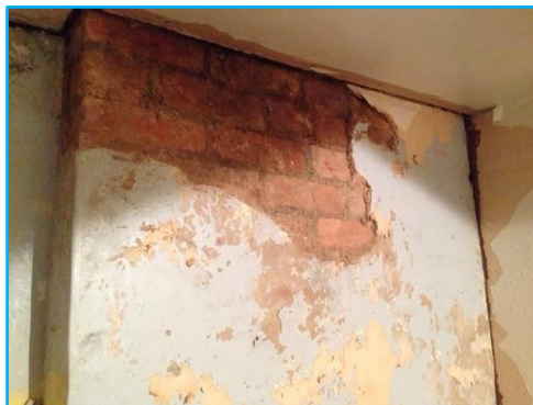
Figure 5. Falling off Plaster found in Walls
