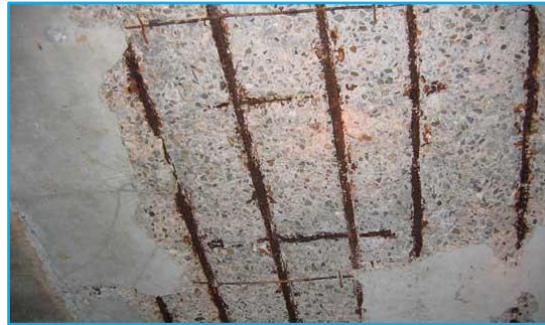
Figure 1. Spalling of roofs
