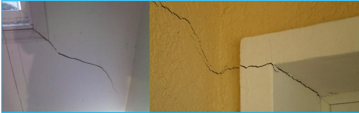
Figure 3. Structural cracks found in doors and windows
