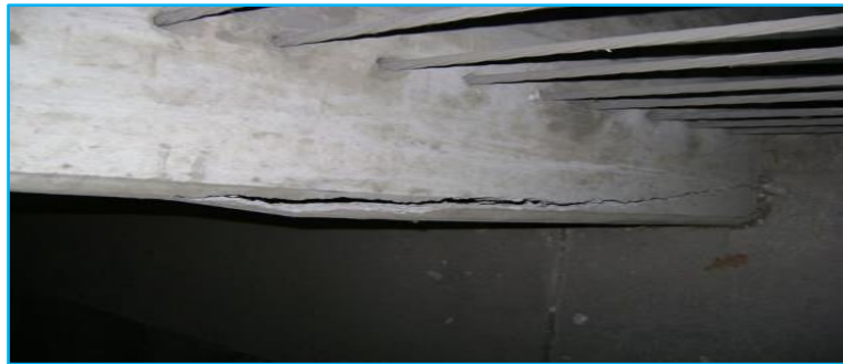
Figure 4. Cracks found in Beams due to excessive loading
