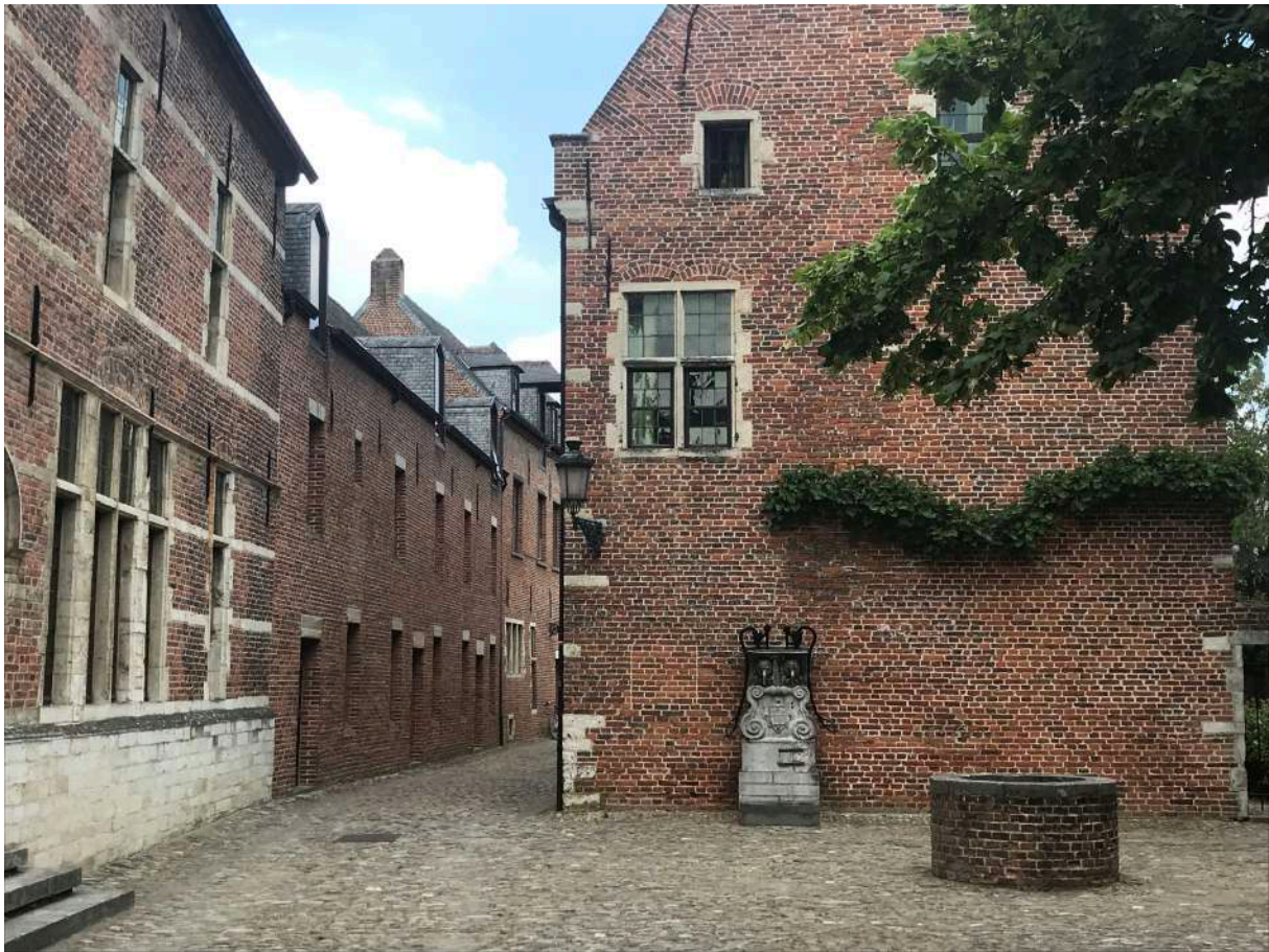
Fig. 2: Louvain, Great Beguinage, View of Benedenstraat after rehabilitation by R.M. Lemaire, ARML.
