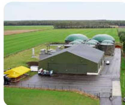
Bio Co-Generation Plant
