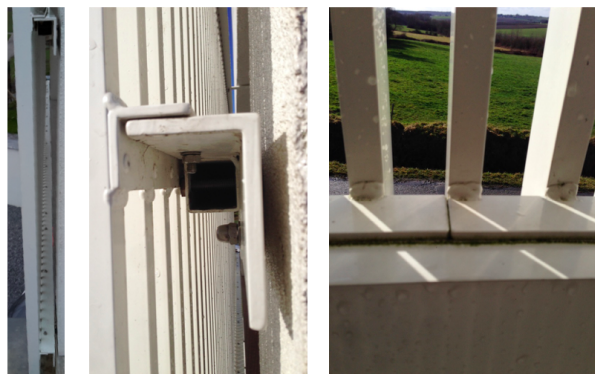
Figure C.1 – Real view on site of cylinders fixation
