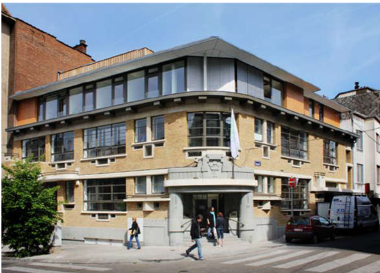
Appendix 2 : Picture of the retrofitted building (A2M 2011).
