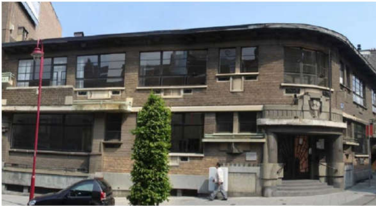
Appendix 1 – picture of the building before refurbishment (A2M, 2011)
