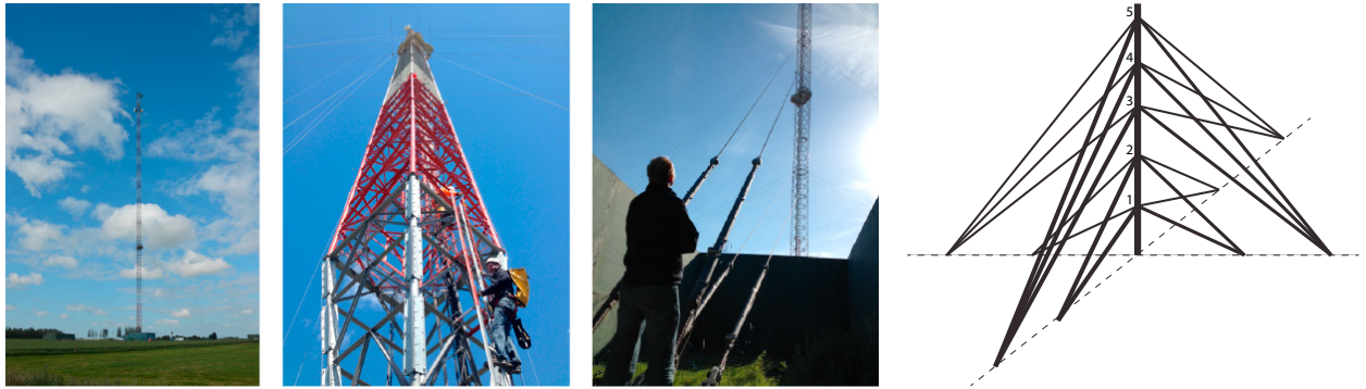
Fig. 1. Schematic representation and pictures of the pylon with the four sets of stay cables, connected at five different levels.
