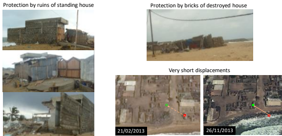
All these 'measures' are temporary and allow at the best to gain a few months
