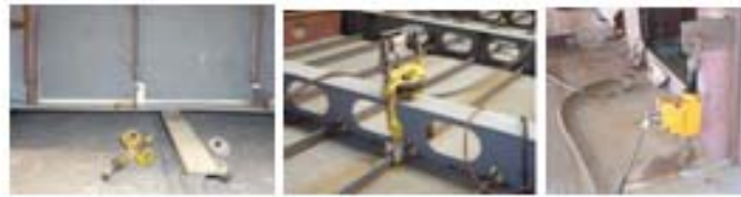
Figure 9 : tools for steel working operations
