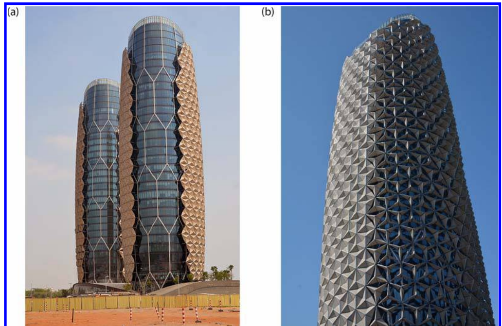
Figure 1. (a) Northern facade and (b) south facade of Al Bahr Towers, with some opened and closed shading devices – coordinates: 24^{\circ} 27' 23'' N, 54^{\circ} 24' 4'' E; alt: 3m (photo courtesy: Terry Boake).
