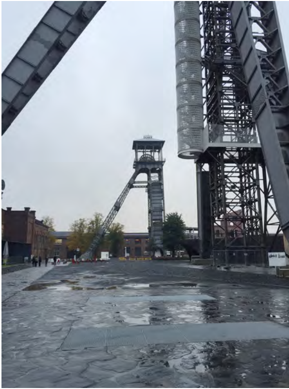
FIG. 1. C-Mine Cultural Centre, Genk, Belgium (by Architects 51N4E). A collection of new developments and adapted buildings is situated around the perfectly preserved pit-head winding gear.
