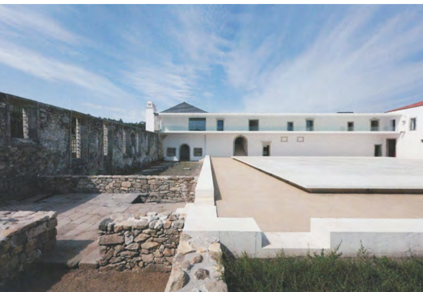
FIG. 8. Mosteiro de Tibães, new building (photo by L. Ferreira Alves).
