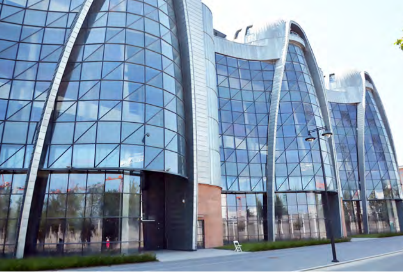
FIG. 15. A new part, designed by Polish architects from MTT Architecture Group, was added to a renovated historical building of EC1 power plant (photo by J. Sowińska-Heim).
