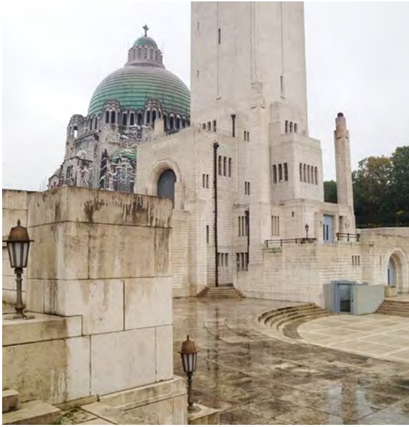
FIG. 1. The Interallied Monument. Exterior (photo by E. Sorbo).
