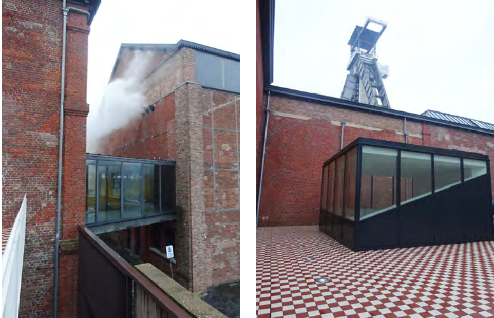
FIGS. 3-4. C-Mine: intelligent and discerning restoration and repurposing.
