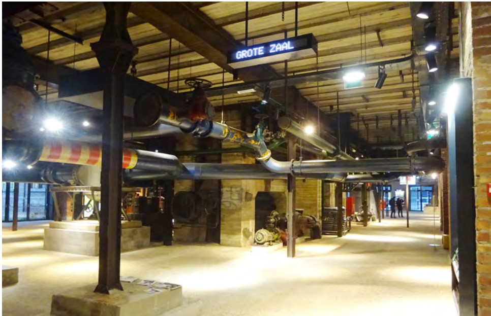
FIGS. 6-7. C-Mine: use of redundant machinery as spatial elements.
