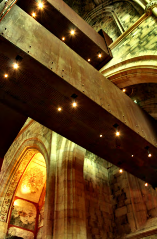
FIG. 7. Maastricht, former church of the Crusaders, Kruissherenhotel; the new connections with the church resulted in new openings breaching and transversing the chapels (by https://www.designhotels.com/hotels/netherlands/maastricht/kruissherenhotel-maastricht [Accessed 19 June 2017]).
