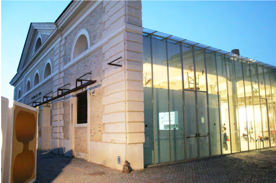
FIGS. 13-14. Rome. The area of 'Mattatoio' in Testaccio reused as a cultural place.
