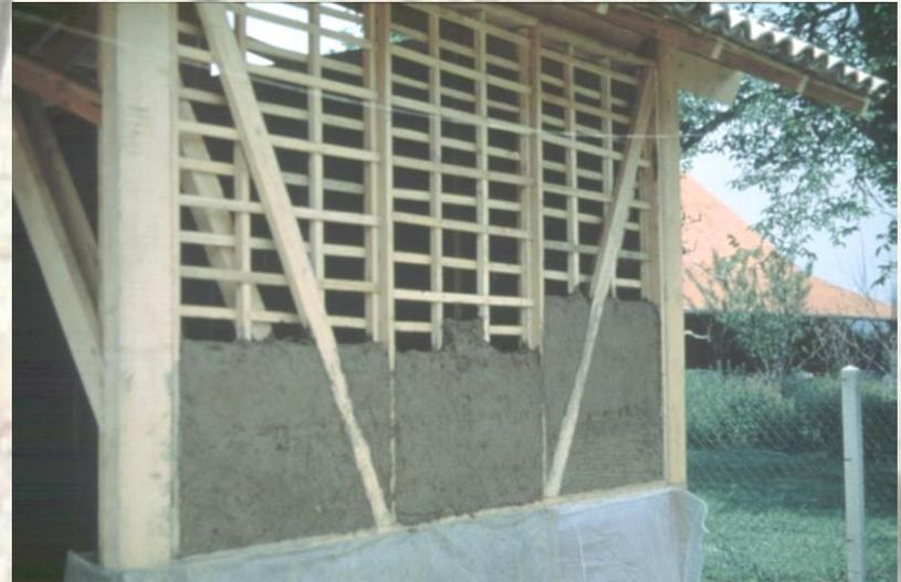
**Wattle and daub**, the earth used in filling load-bearing structures, usually made of wood.
