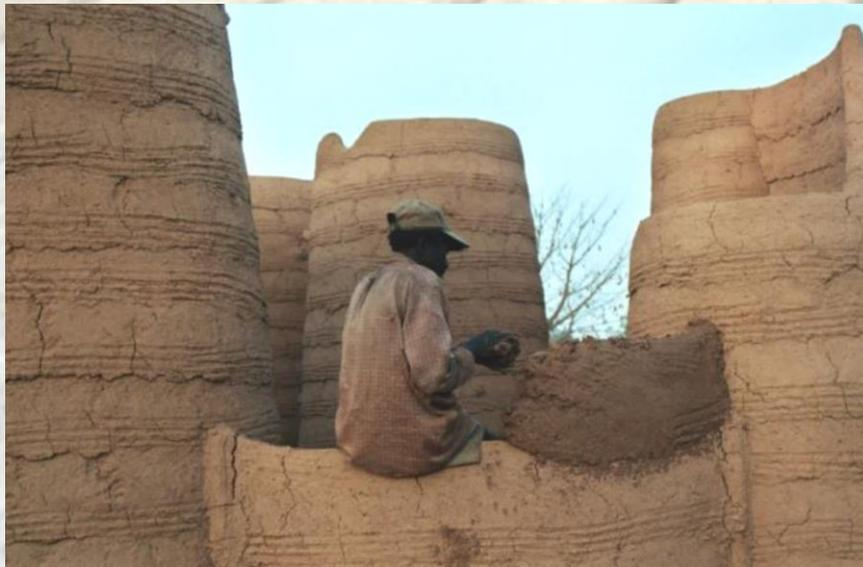
**Cob**, the earth built in layers
