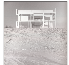
House II_1969 front view
