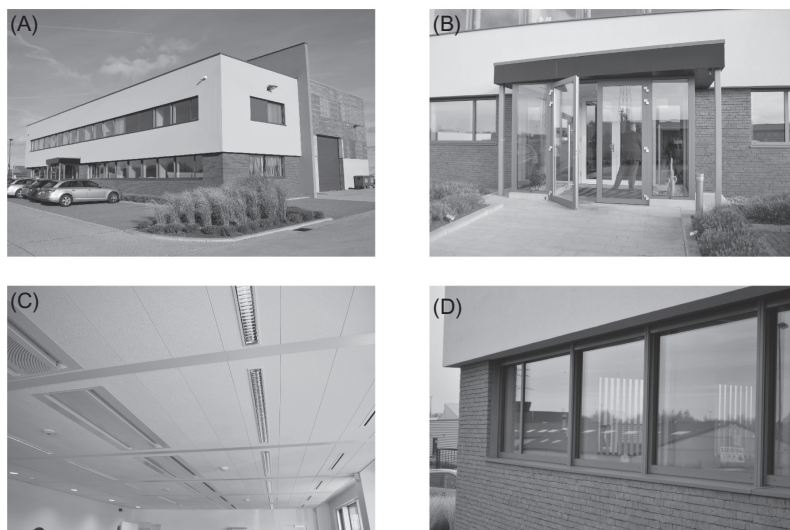
FIGURE 11.5 (A) The office building in the front and factory in the back, (B) the main building entry and the security airlock system, (C) the ultra-efficient LED tubes and the linear ventilation supply in the center and exhaust on the side of the office space, and (D) the external automated shading blinds for solar protection.
