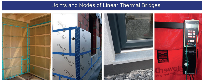
FIGURE 9.5 Joints and nodes of linear thermal bridges (Architecture et climat).
