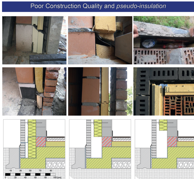
FIGURE 9.2 Examples of poor construction quality and pseudo-insulation (Staepels et al., 2013).
