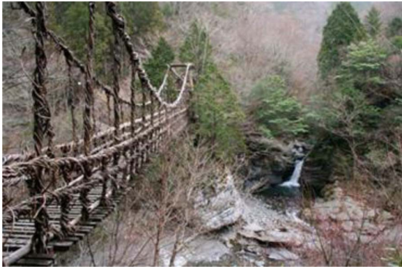
Figure 1 Vine bridge in the Iya Valley, Japan (photo from Funzug.com ).
