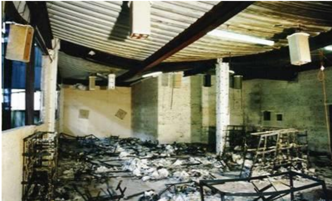
Cardington fire test, UK, 1997
