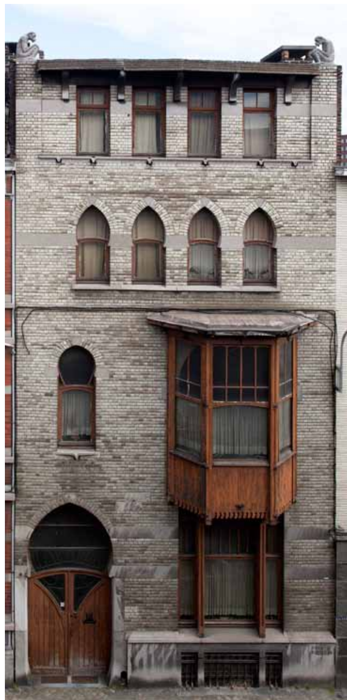
In the Van der Schrick House (1906–1906), Paul Jaspar experimented with new materials like concrete. Left, detail of acroterion atop the house made by Oscar Berchmans
