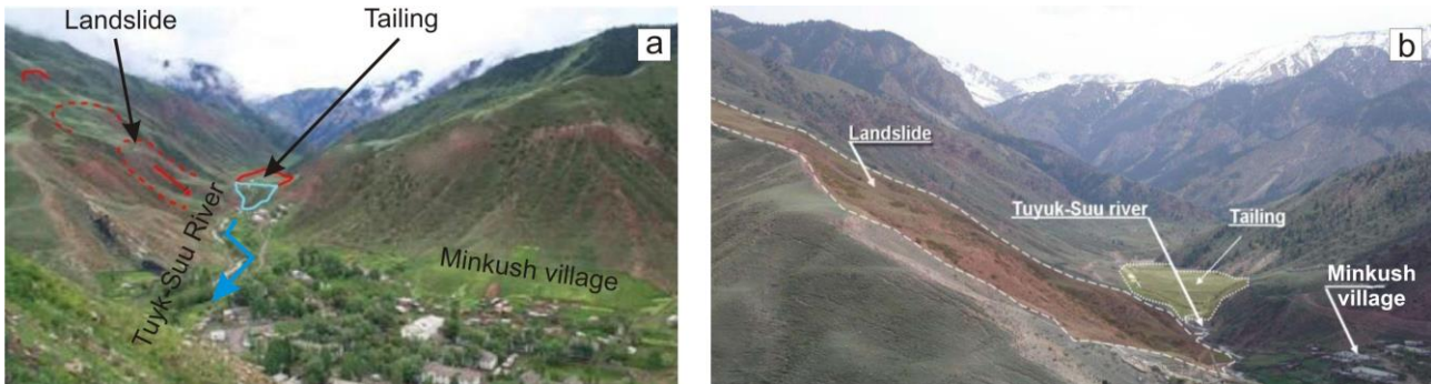
Figure BF.82: Views of the Tuyuk-Suu tailing, landslide and the Minkush village showing the high exposure of the tailing site to potential impacts of the landslide activity.
