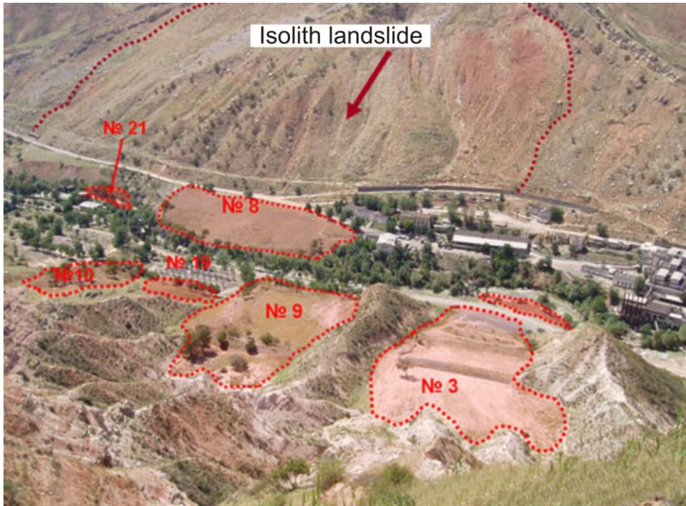
Figure AF.26: The radioactive tailings (red dotted outlines) situated in a narrow river valley, subjected to the negative impacts of the landslide activity (the courtesy of the Ministry of Emergency Situations Agency of Kyrgyzstan)
