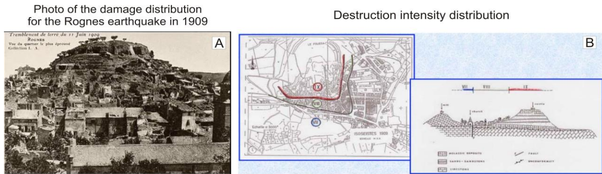
Figure BF.6: (a) Photograph showing the damage distribution caused by the Rognes earthquake in 1909 showing a more intense destruction close to the crest of the hill; (b) sketch of the seismic intensity distribution indicating higher level of destruction in the topographically high areas (by Bard, 2007).
