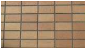
Fig. 28/29/30/31/32/33- Facades' details. Tiles cladding - Kamisaginomiya - Tokyo. (Photo by the Author)
