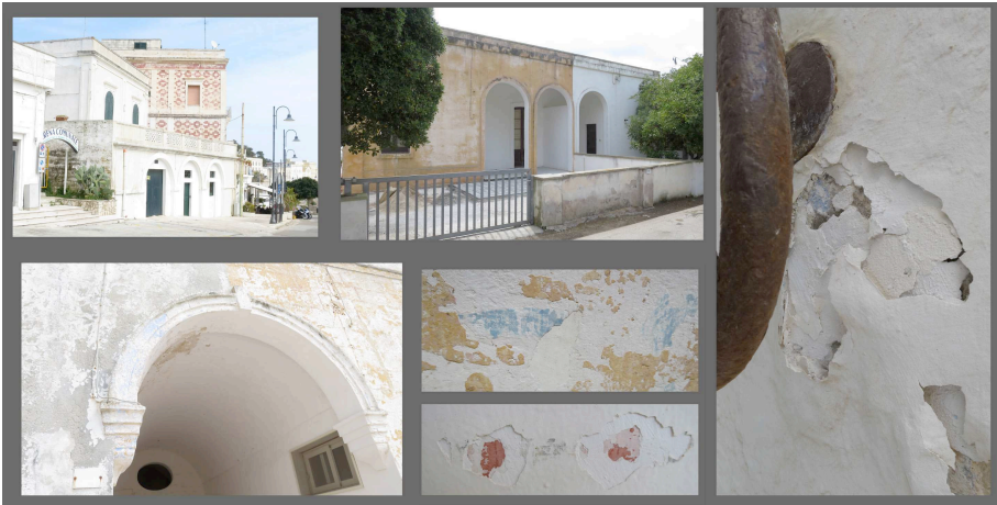
Fig. 10 – Santa Cesarea Terme: bright colours resurfacing from whitish superficial layers on exterior and interior facades.
