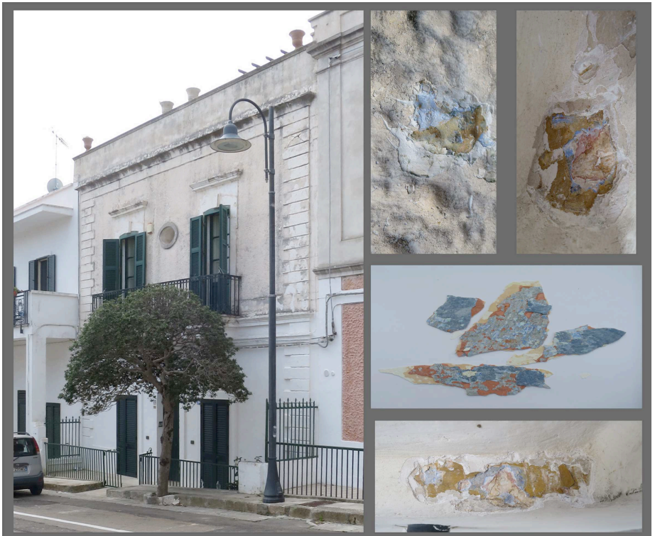
Fig. 11 – Santa Cesarea Terme, via Piave: a white facade originally characterised by a series of coloured architectural elements (basement, cornices, ashlar work).
