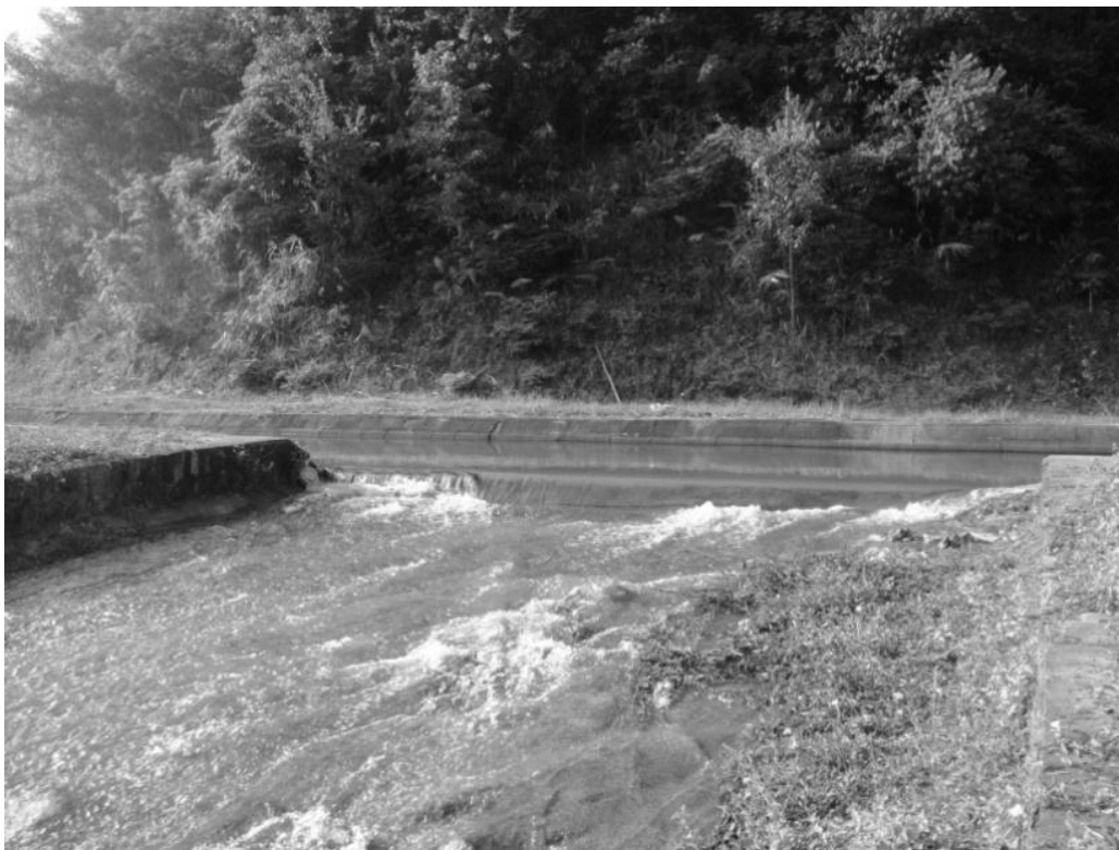
Photo 2. Second drop on the concrete channel for water releases to Nam Nyam in rainy season (Namnyam, August 2010).
