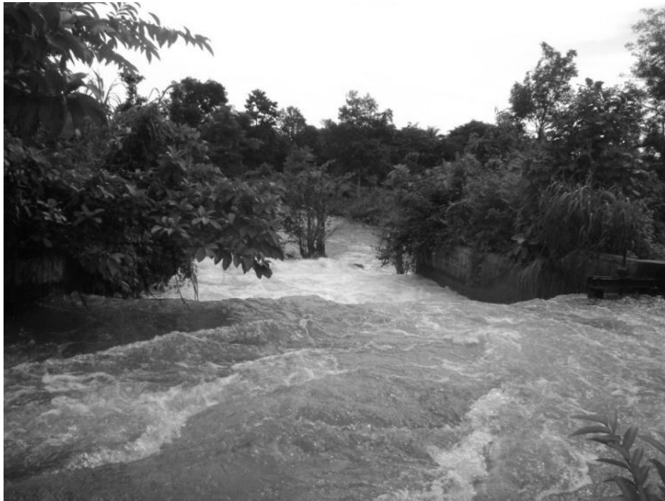
Photo 1. First drop on the concrete channel for water releases to That Nam Dan waterfall and Nam Teng in dry season. (Namnyam, May 2012)
