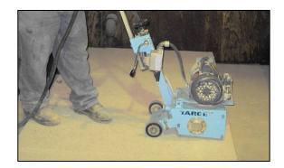
Figure 3-5: Scarification and shotblasting surface preparation at CRIB (UL program)
