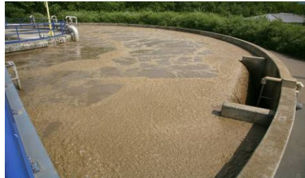
Biological treatment Activated sludge reactor
