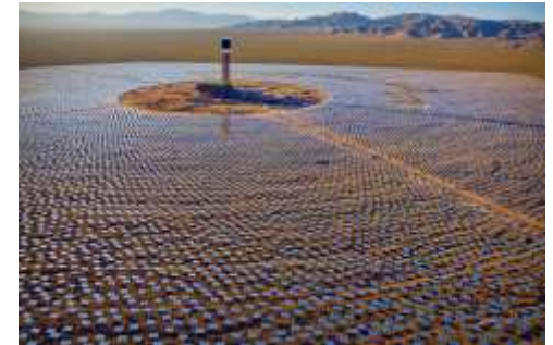
Ivanpah CSP plant (392 MWe)
