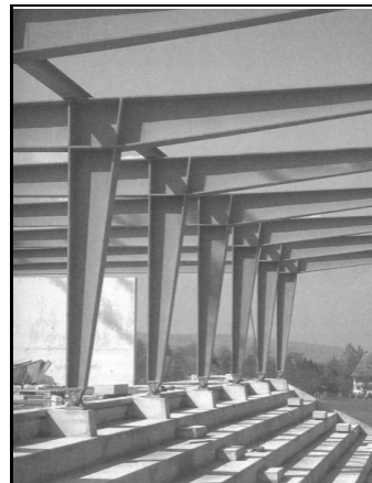
Figure 1: tapered section elements.
