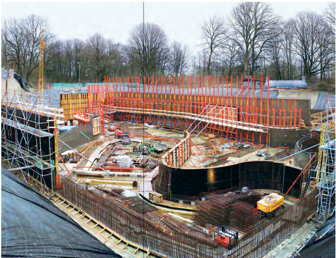
3a-c The trajectory of the curves during the design process: from contour lines on the plan given to the architect to poured concrete walls on the construction site.
