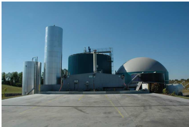
Figure 16: Picture of the plant “Biogasyll”.
