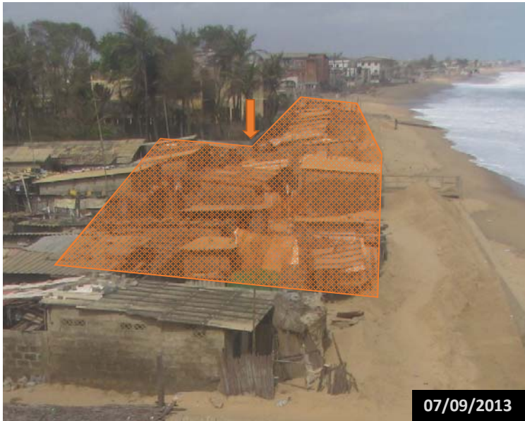
Makeshift houses destroyed by the sea in 24h (30-31 May 2014)
