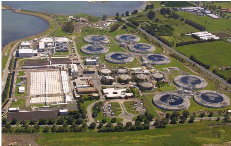
Figure 3. Water treatment plant
