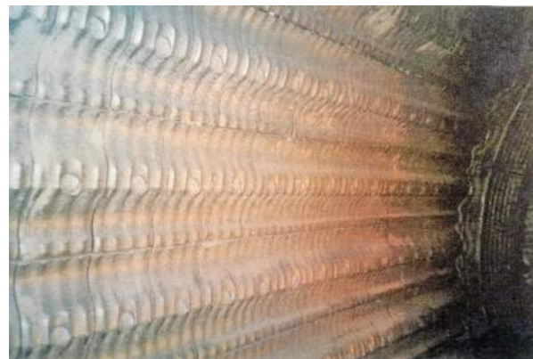
(b) Liner plates along the first compartment.
