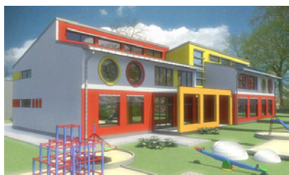
Figure 5 – The Sun kindergarten in Gabrovo – the first passive public building in the country: (source: Passive House Buildings , 2013)
