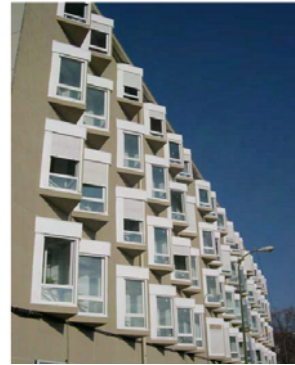
Figure 13 – Renovated building – East façade
