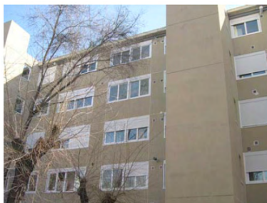
Figure 15 – Rehabilitated building – West façades
