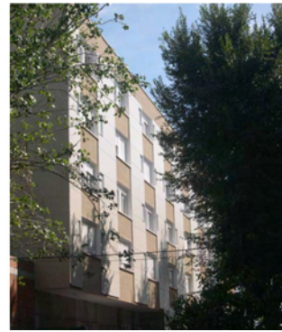
Figure 12 – New building – West façade
