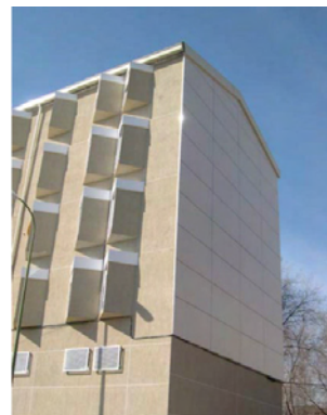
Figure 14 – Rehabilitated building – North and East façades
