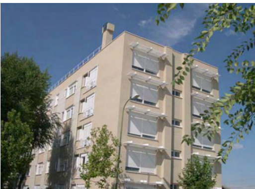
Figure 11 – New building – South façade
