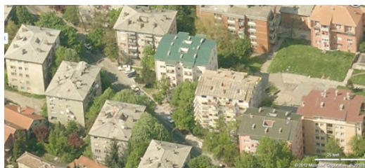
Figure 10 – Buildings in Vojvode Micka Street, Karaburma, bird's eye view
