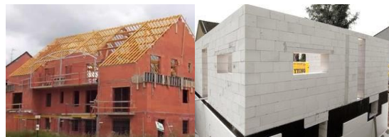
Figure 1. Multi-storey apartments (left) and lightweight concrete house (right)
