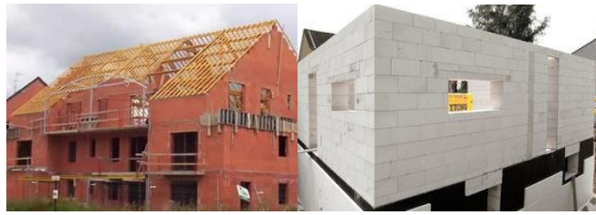
Figure 1. Multi-storey apartments (left) and lightweight concrete house (right)
