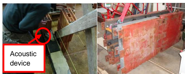
Figure 5. Sound proofing devices and additional mass
