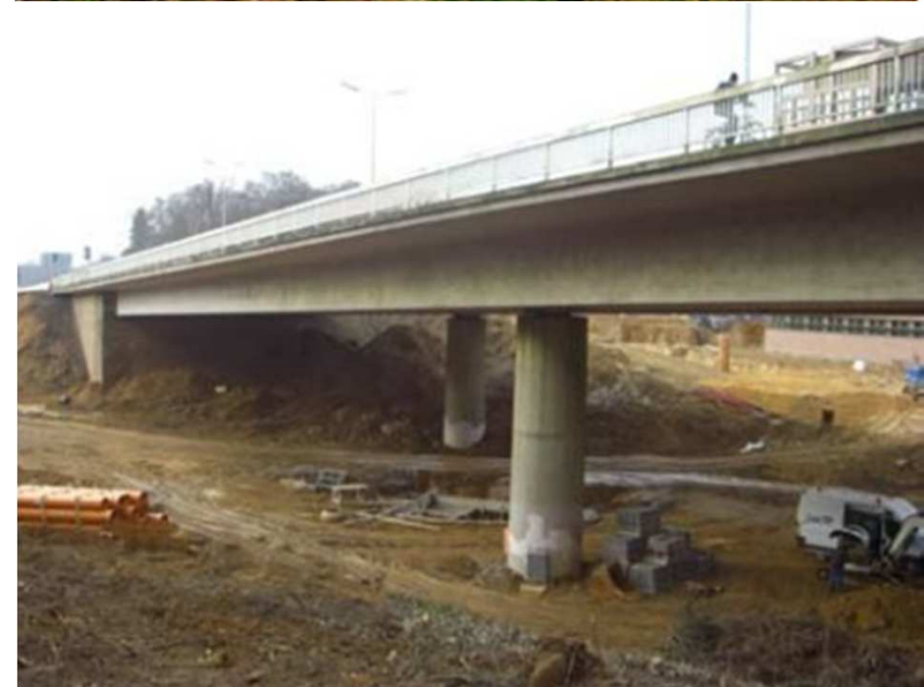
Views of the Champangshiehl bridge (Luxembourg)
