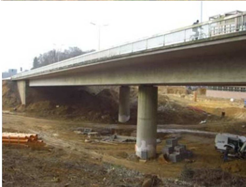
Views of the Champangshiehl bridge (Luxembourg)
