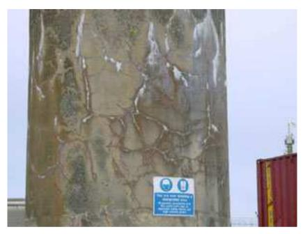
Habour installation from the 1970's containing Diorite and granites with opaline veining coarse and fine aggregate (BRE-UK).
