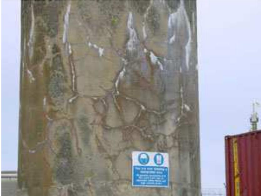
*Harbour installation from the 1970's containing Diorite and granites with opaline veining coarse and fine aggregate (BRE-UK).*
