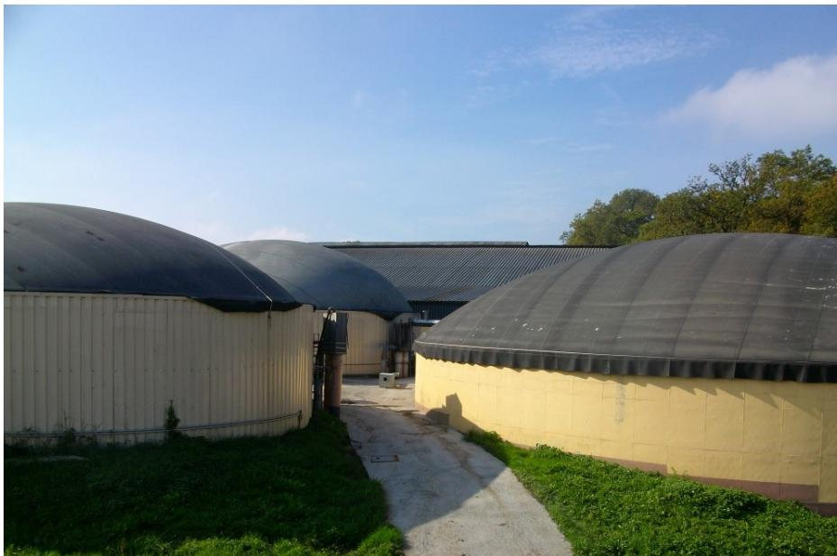
**Co-digestion biogas plant of 750 kW
