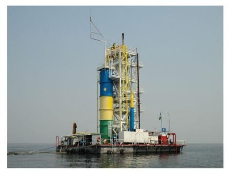
**Fig. 1.4** Gas extraction facility of Kibuye Power 1 (KP1), the first pilot plant for large-scale commercial methane extraction from Lake Kivu that started operating in January 2009 (Photo provided by Kibuye Power Ltd.)
