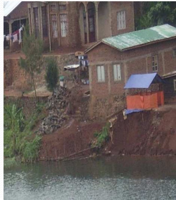
Figure 11: Landslide after the earthquake of 03/02/2008
