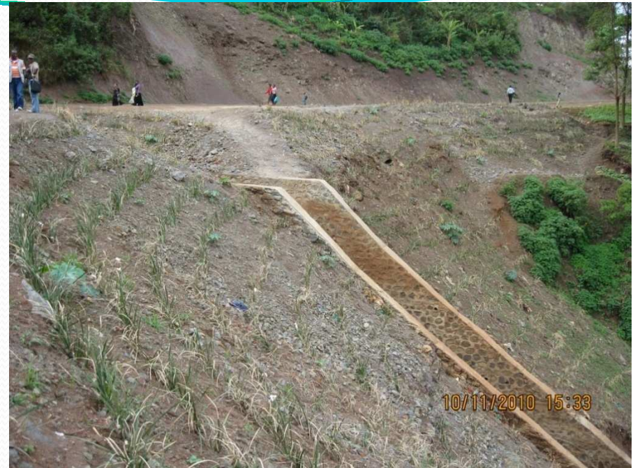
Drainage and slope stabilization in Bukavu
