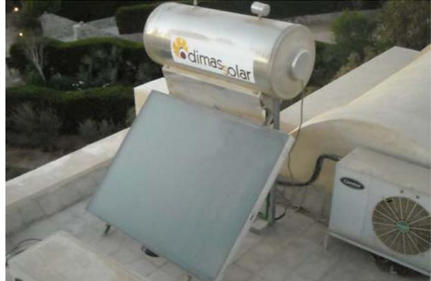
Fig. 6: Dimas Solar Thermosyphon installed on the roof
