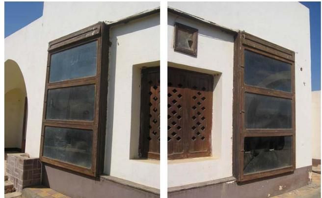
Fig. 3: The Trombe wall system with southern exposure
