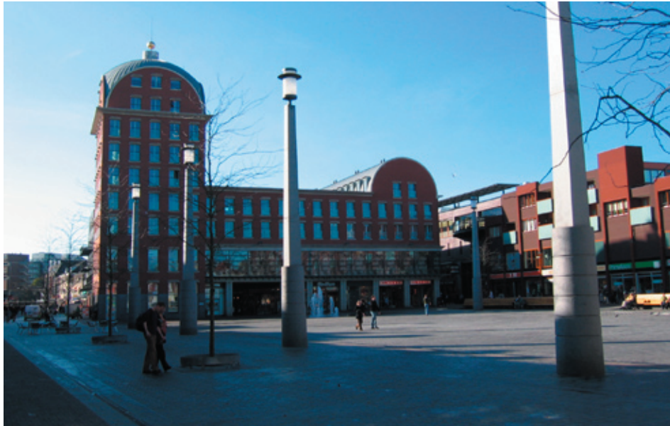
Fig. 3.14, V&D Building, Statenplein
