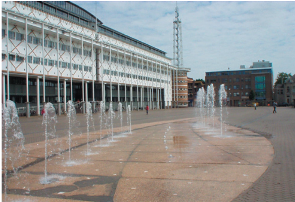
Fig. 3.30, The Municipality building and the fountain
