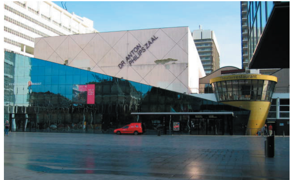
Fig. 3.59, The eastern side of Spuiplein
