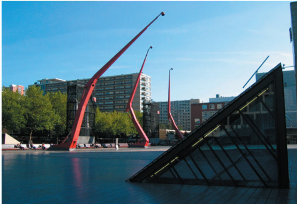
Fig. 3.08, Triangular glass prism for garage exit, Schouwburgplein
