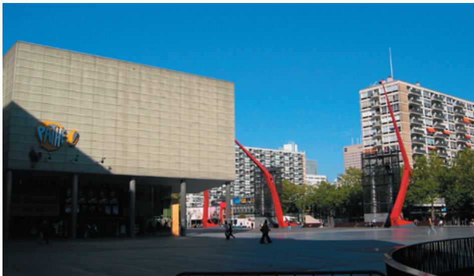
Fig. 3.09, Schouwburg plein and Cinema Building
