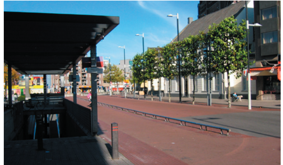
Fig. 3.05, Red asphalt bus lane
