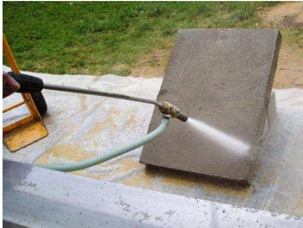
Figure 20 : Concrete slabs sandblasting operations
