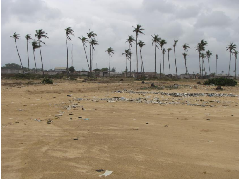
Cotonou: shoreline erosion – RESPONSE (2013-09)
