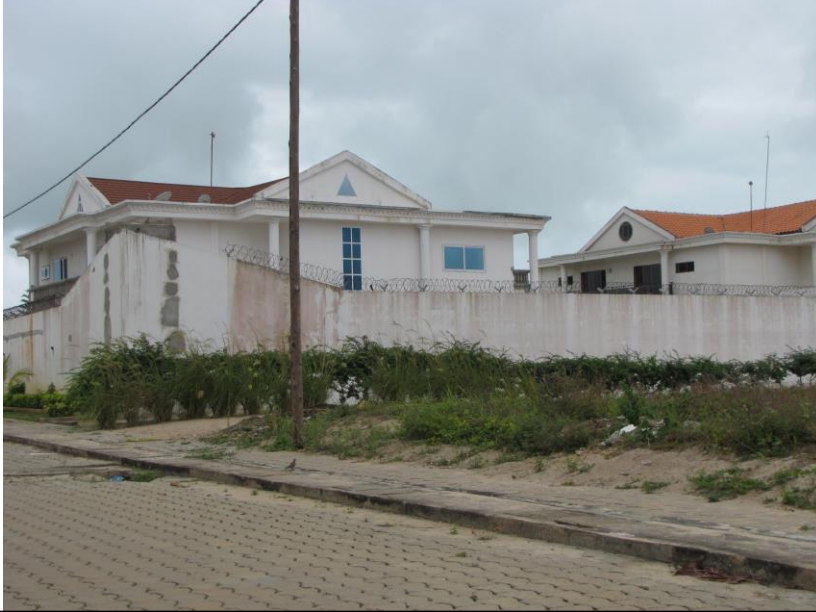
Cotonou: shoreline erosion – RESPONSE (2013-09)
