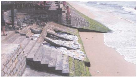
Fig. 10: Seawalls destroyed by erosion processes at the limit of the western resorts (For location, see: Fig. 3 [c])
