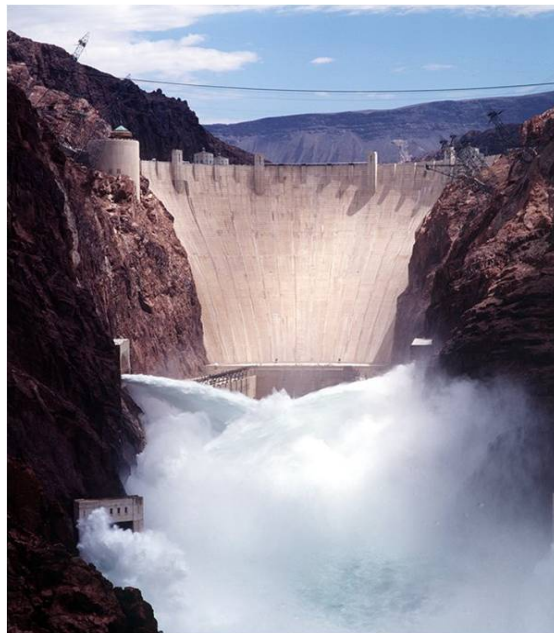
Figure 5.30: Impacting jets from the Hoover dam (source: United States Bureau of Reclamation)
