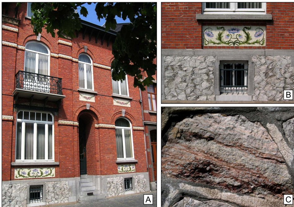
Figure 16. A–C. Lower part of 20th century middle-class house (Art Nouveau style) with substructure made of irregular blocks (B) of grey and pink Marble of Baelen. C. Detail of irregular block showing contact between red-stained “pierre poitée” facies (below) and pink stromatactis-bearing limestone (above). Hasselt, Guffenslaan n°100.
