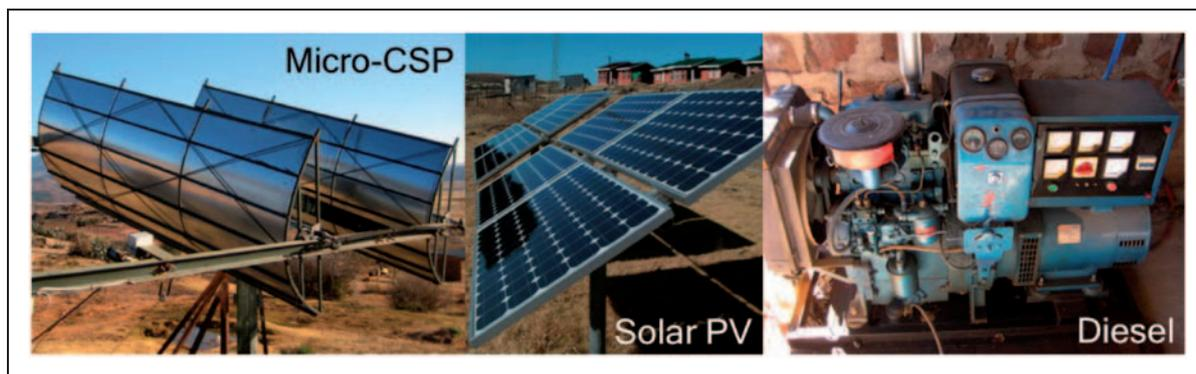
**Figure 1.** Three technologies for generating electricity at remote mini-grids:  $\mu$ -CSP (concentrating solar power), solar photovoltaic (PV) panels, and diesel generators.  $\mu$ -CSP, a solar thermal technology, is also configurable to deliver combined heating and power (CHP).
