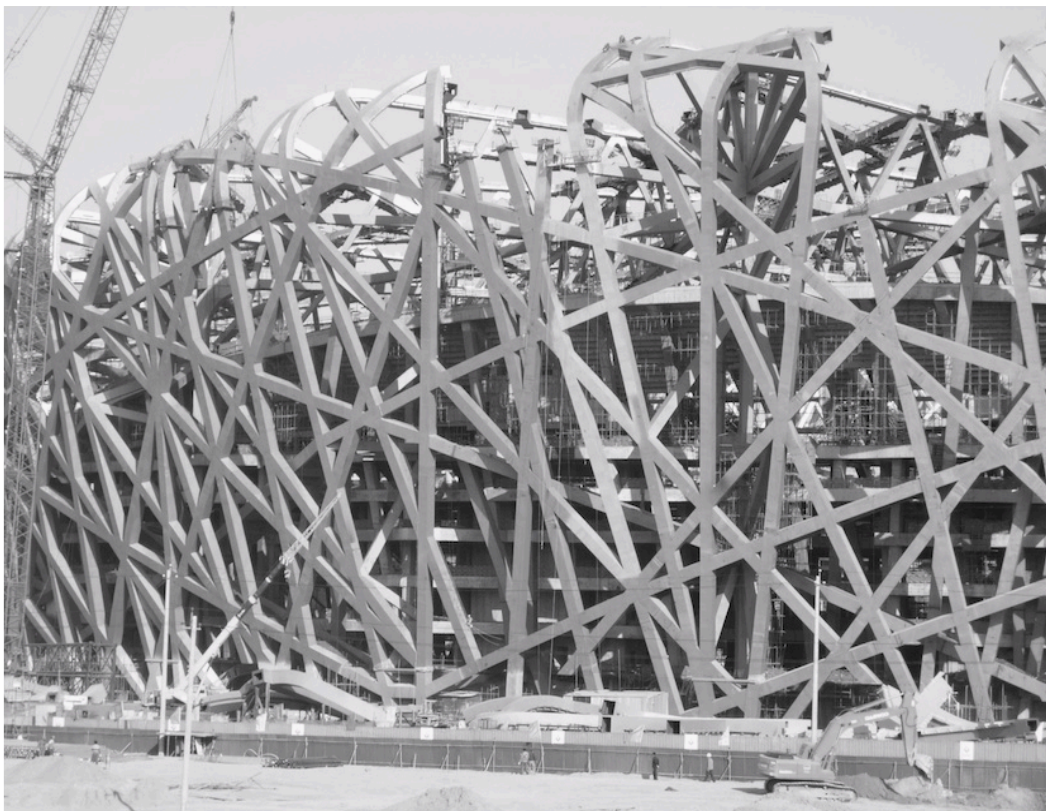
Figure 2: Beijing Olympic Stadium construction (2006) (Source: Miranda Kiuri).
