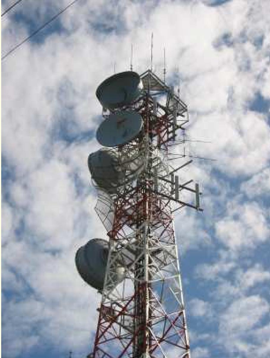
FIGURE 9.9 – Exemple d'antennes paraboliques (ROCKHAMPTON, QUEENSLAND, AUSTRALIE).
